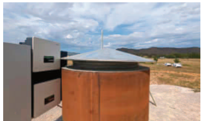
Above Ground Installation
